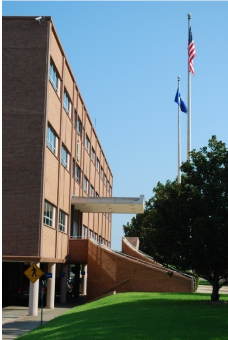
Photo 8. The former Shreveport City Hall rests on pilotis, making it appear to float above the ground. Note the strong geometry in the entrance, which is skewed to one side.
